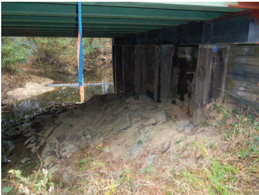
Photograph No. 8: View looking west along End Bent 2
