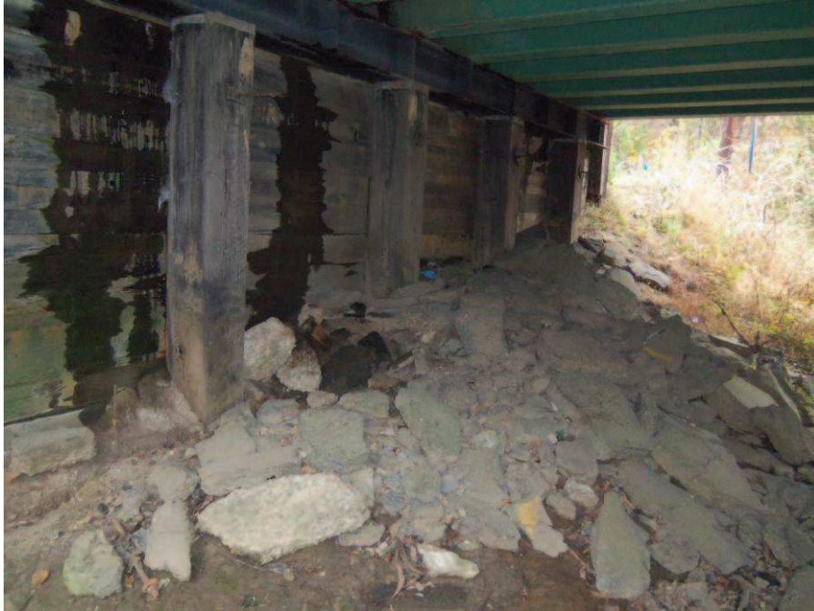
Photograph No. 7: View looking east along End Bent 2
