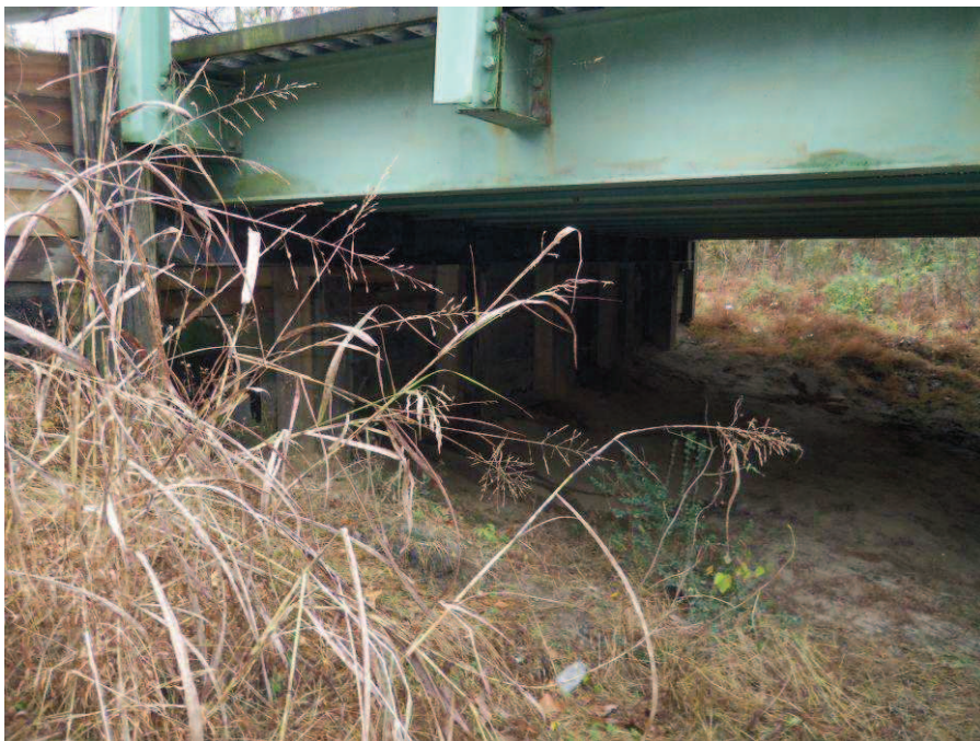
Photograph No. 6: View looking west along End Bent 1
