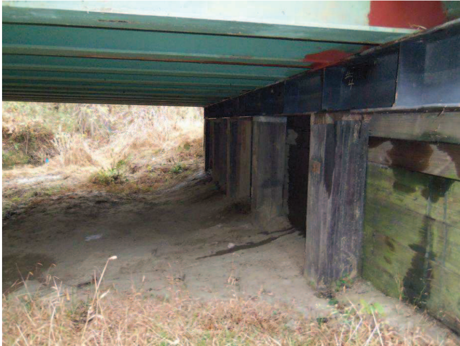
Photograph No. 5: View looking east along End Bent 1
